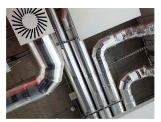
Kingspan Kooltherm™ FM Pipe and Duct Insulation have been assigned a highest possible 2008 Green Guide Summary Rating of A+ by the BRE. Kingspan Kooltherm™ FM Pipe Insulation has also and has been awarded a best-in-class Eurofins Indoor Air Comfort Gold certificate, recognising it as outstanding material according to the VOC Indoor Air Quality emissions standards. Kingspan Kooltherm™ FM Pipe Insulation is the first pipe insulation product to attain BDA Agrement® certification under the scheme.
